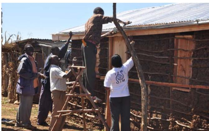
The three-roomed shelters under the ADB funding include fascia boards and provide support for gutters to channel rainwater into 500 plastic water tanks.
